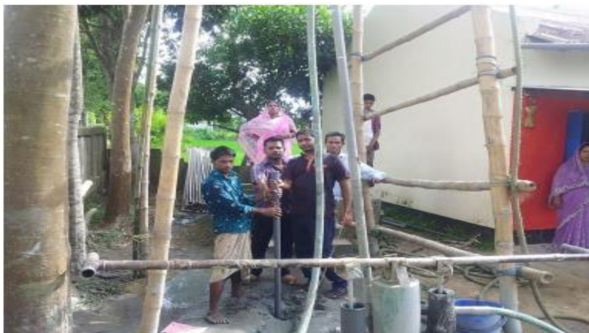
Fig. 13 Lowering of Tube well in presence of school authority
