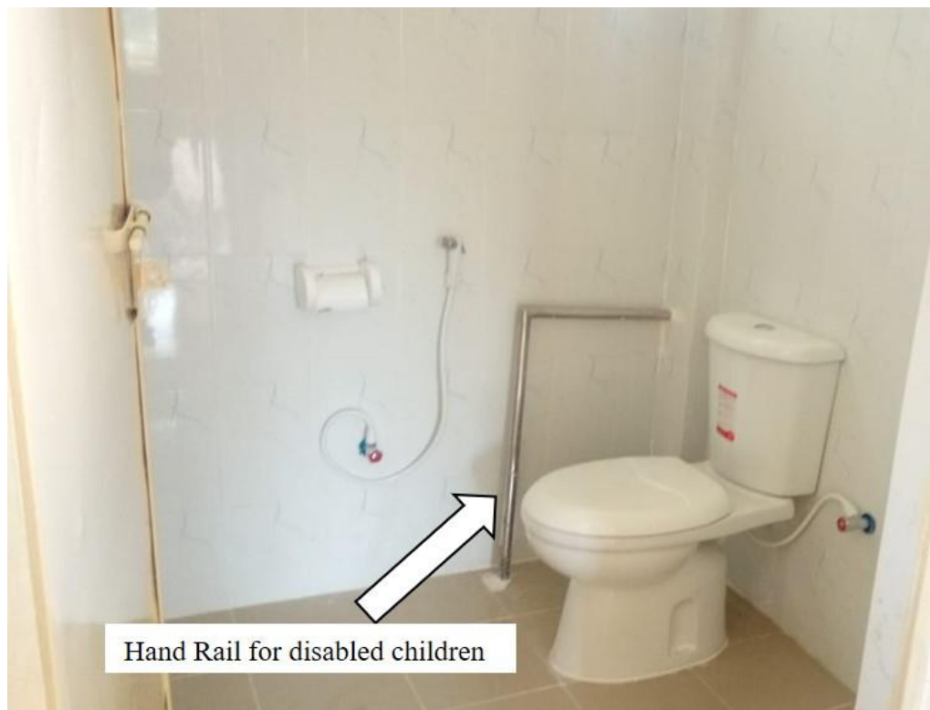
Fig. 10 Toilet for disabled children
